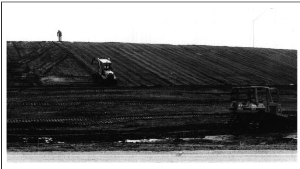
Figure 2.3 Application Of Mulch/Soil Mix On Slope
