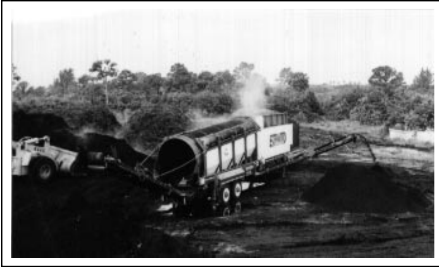
Figure 7.5 Trommel Screen
