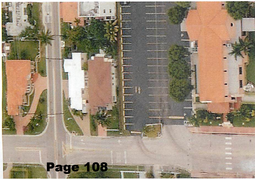
EXISTING CONDITIONS - BIRD'S-EYE-VIEW, FACING SOUTH
