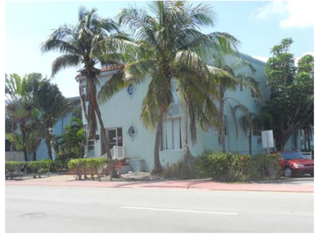
View showing the north façade and continuous roofline banding, March 2014.
