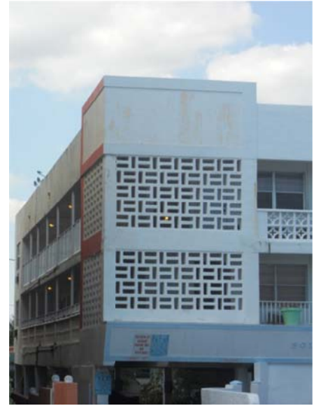
Detail of the brise-soleil patterns, March 2014.
