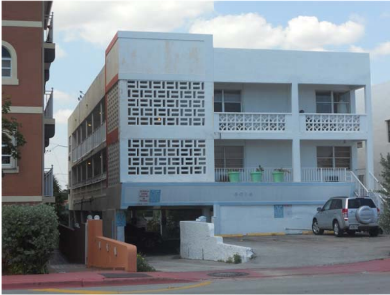
The main and south façades of 9016 Collins Avenue, March 2014.
