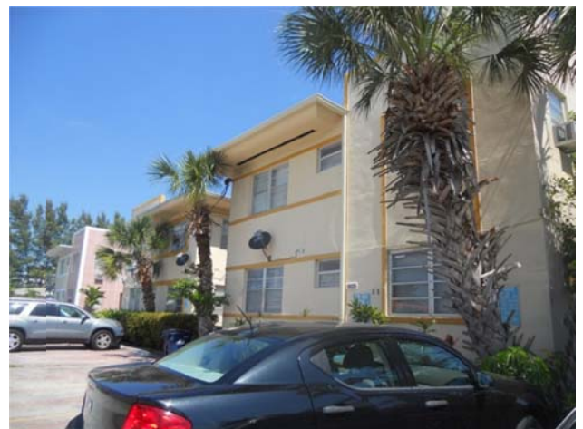
View looking northeast from Harding Avenue of the grouping of three nearly identical MiMo buildings, March 2014.
