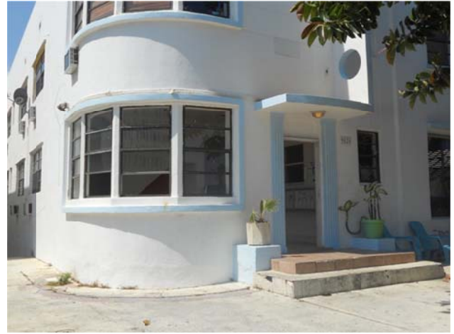
View of the entry details and first floor of the rounded corner, March 2014.
