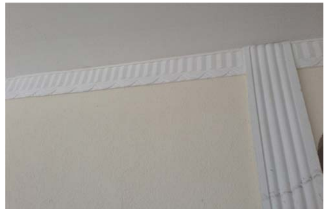
Detail of the interior lobby, March 2014.
