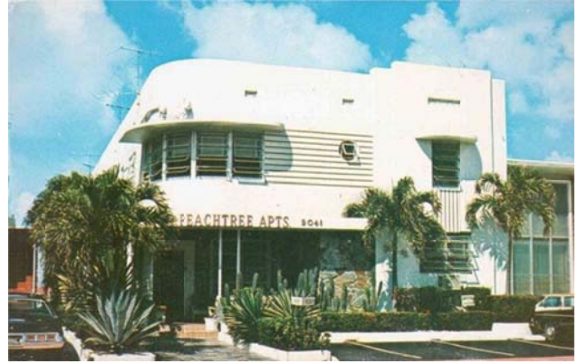
Historic period photograph of Peachtree Apartments showing the widened first-floor windows on the façade, circa 1960s.
