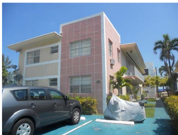
View of the main façade of 9041 Harding Avenue, March 2014.
