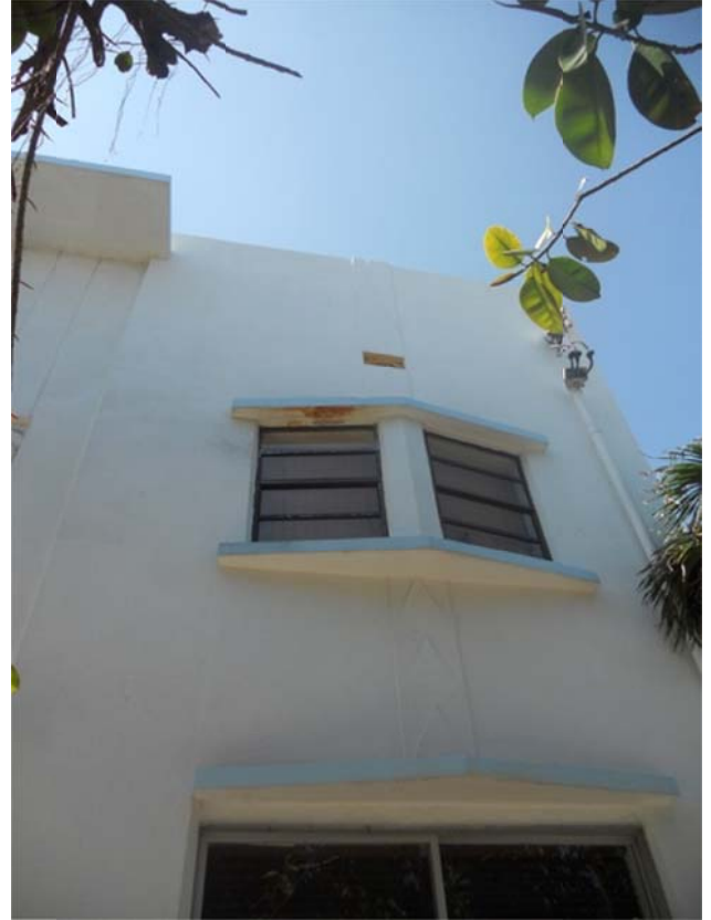
Detail of the third portion of the main façade with triangular eyebrows and geometric banding, March 2014.
