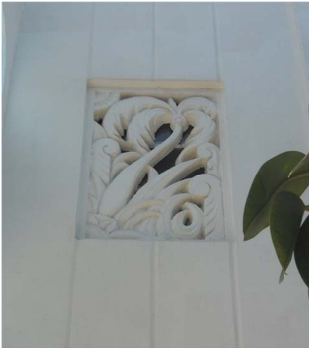
Detail of the tropical concrete block and vertical striations, March 2014.
