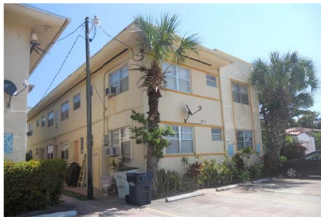
View of the main façade of 9025 Harding Avenue, March 2014.
