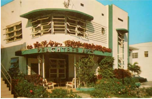
Historic period photograph of Peachtree Apartments showing the original windows on the façade and the widened eyebrow with signage over the entry, 1955.
