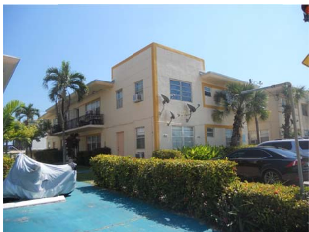
View of the main façade of 9033 Harding Avenue, March 2014.
