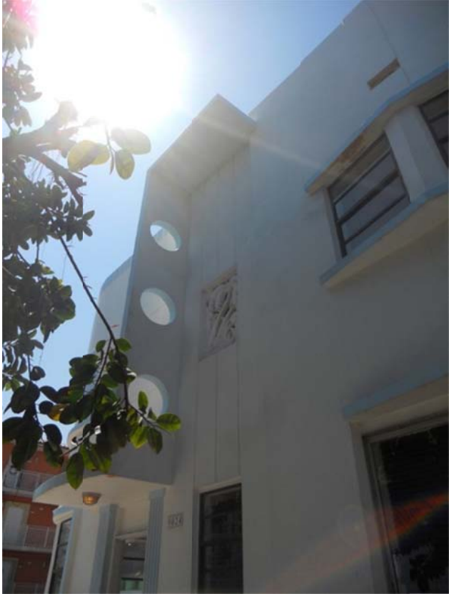
Detail of the tripartite eyebrow, porthole cutouts, and triangular eyebrows, March 2014.
