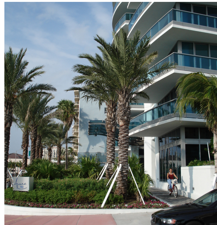
RECENTLY BUILT CONDOS ALONG THE BEACH-FRONT
