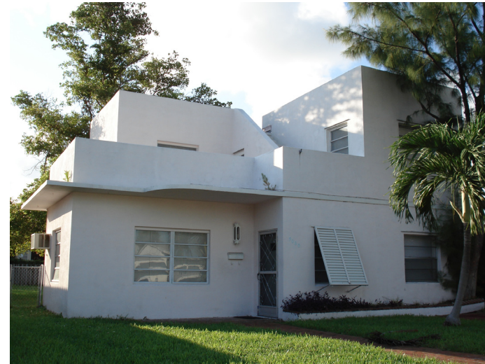
A TYPICAL SMALL SURFSIDE HOUSE IN MODERN STYLE
