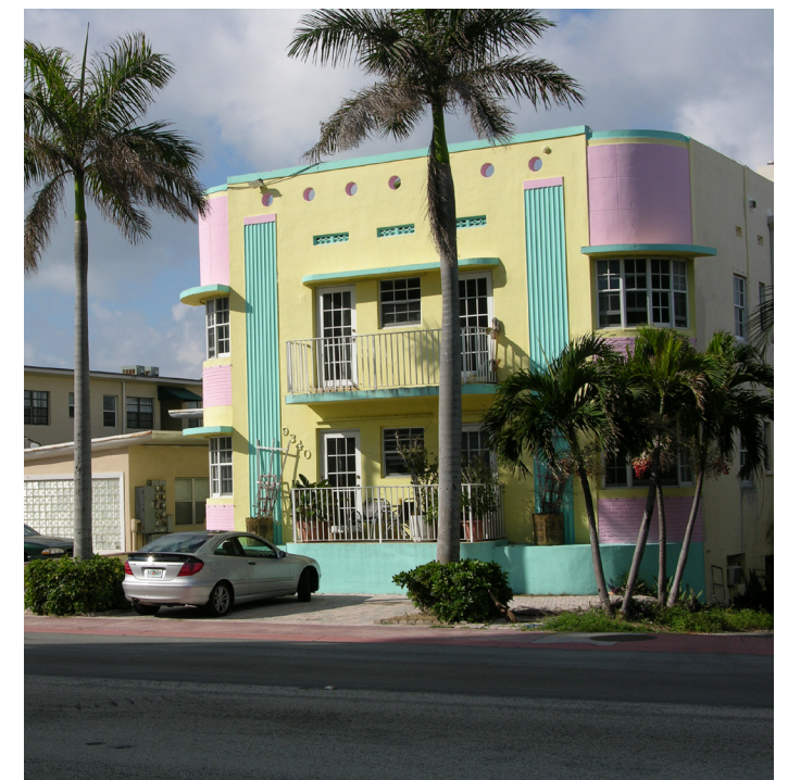
EXISTING ART DECO APARTMENTS ALONG COLLINS AVENUE
