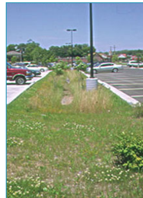
The Discovery Center parking lot features bioswales planted with native species that filter pollutants from parking lot runoff.
