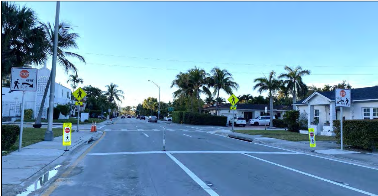
Photograph 1: Looking South - View of SR A1A/Harding Avenue and 89 Street Intersection
