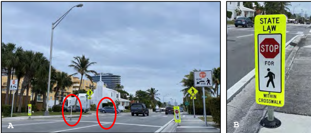
Photograph 5: Missing In-Street Pedestrian Crossing Signs (R1-6a)
