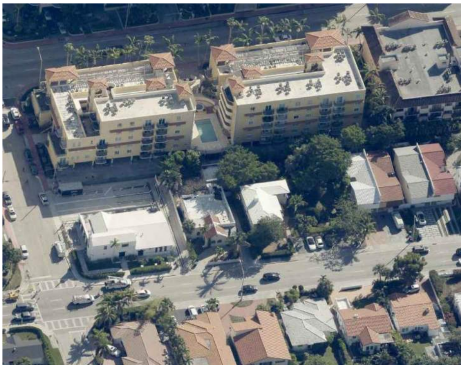
3 EAST AERIAL VIEW (FROM HARDING AVE)
