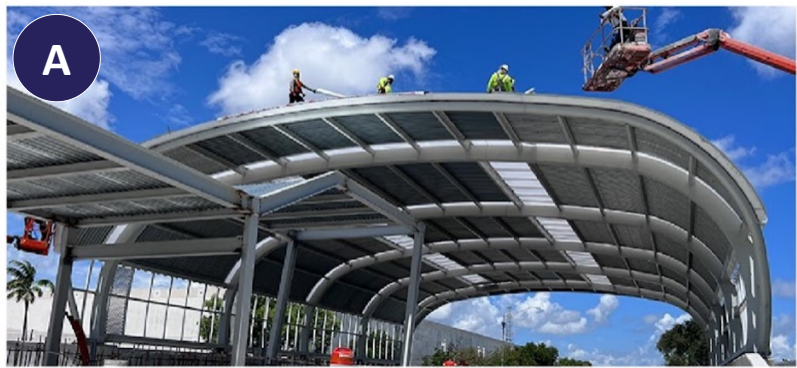
A South Corridor: Bus Transit, under construction
