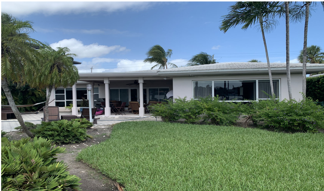
940 88 ST. REAR VIEW
