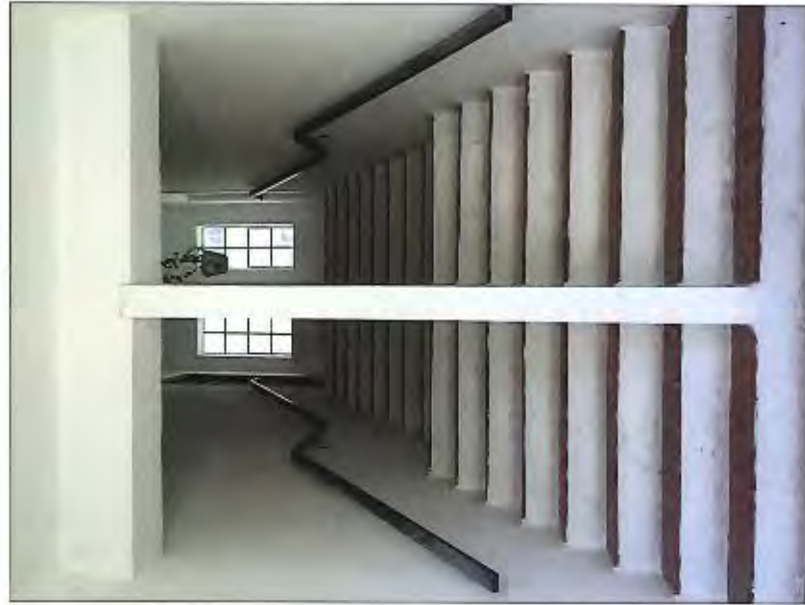
3 STAIRS TO UPPER UNITS
