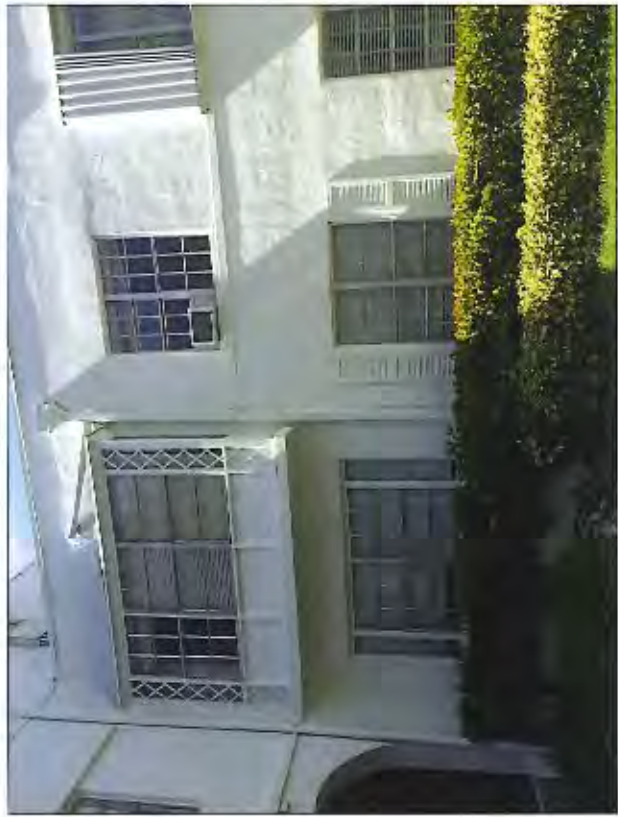
1 NORTH WING APARTMENTS WINDOWS AND VERANDA
