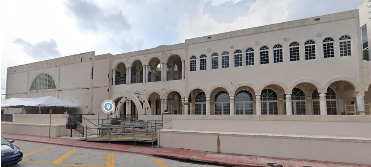
9540 Collins Avenue – Main Synagogue Building - view 2022 / Image courtesy of Google Maps- 2022
