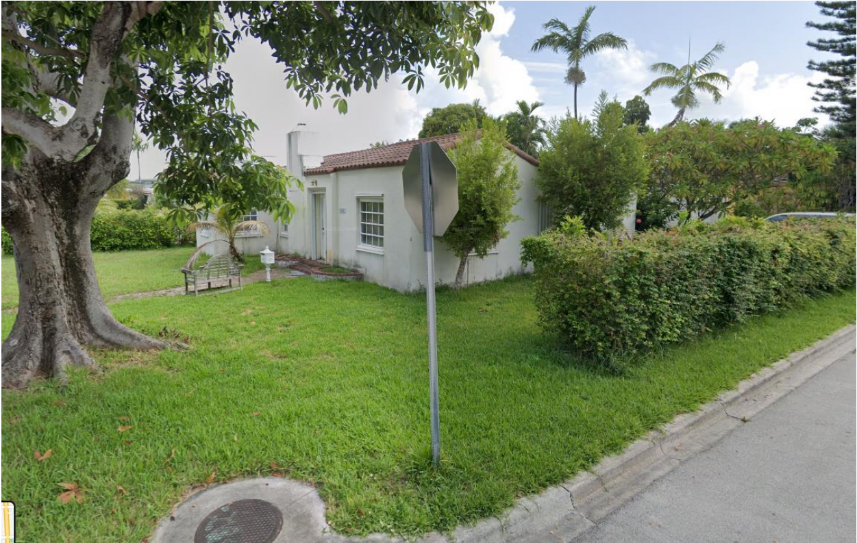
8801 Emerson Avenue, View from 88 th Street / Image courtesy of Google Maps 2022
