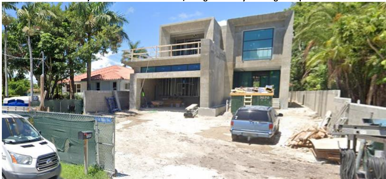
9208 Bay Drive / Image courtesy of Google Maps 2022
