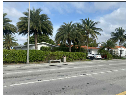
EXISTING NEIGHBOR'S HOUSE
