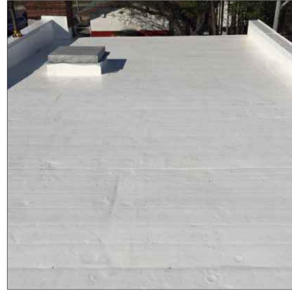
Built-up Roofing (White)
