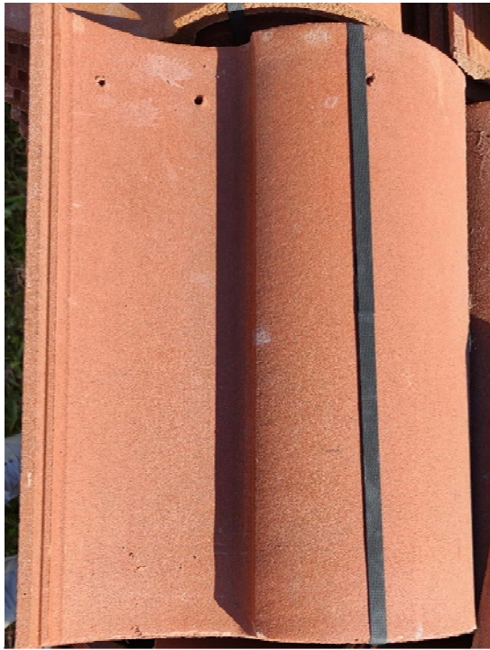
Barrel Tile Roof
