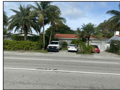
EXISTING NEIGHBOR'S HOUSE
