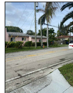
EXISTING NEIGHBOR'S HOUSE
