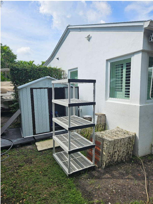
Figures 4-7: North Side of home at 525 95th Street
