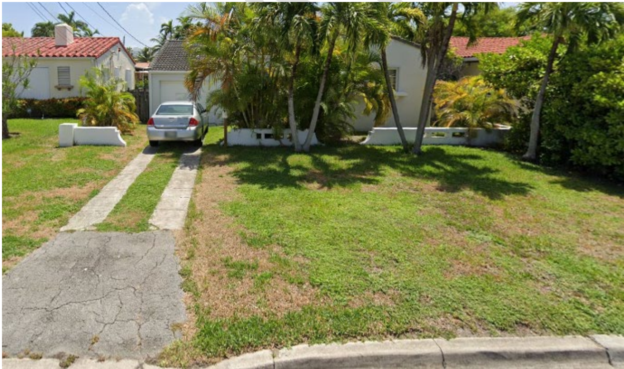
West Elevation of 8935 Froude Avenue
