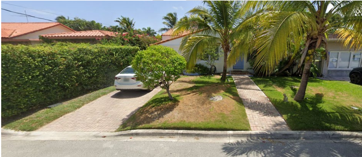
East Elevation of 8841 Garland Avenue
