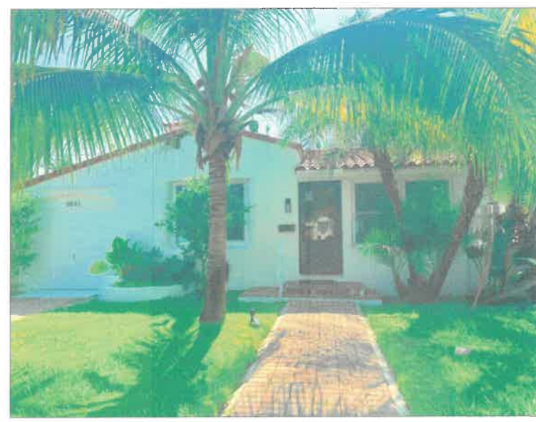
FRONT FACING GARLAND AVENUE
