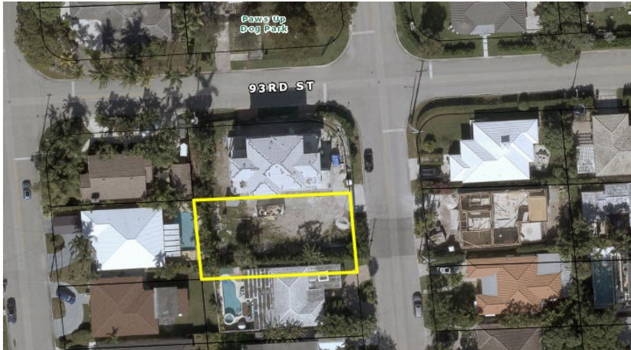
Aerial view of 9280 Byron Avenue under construction
