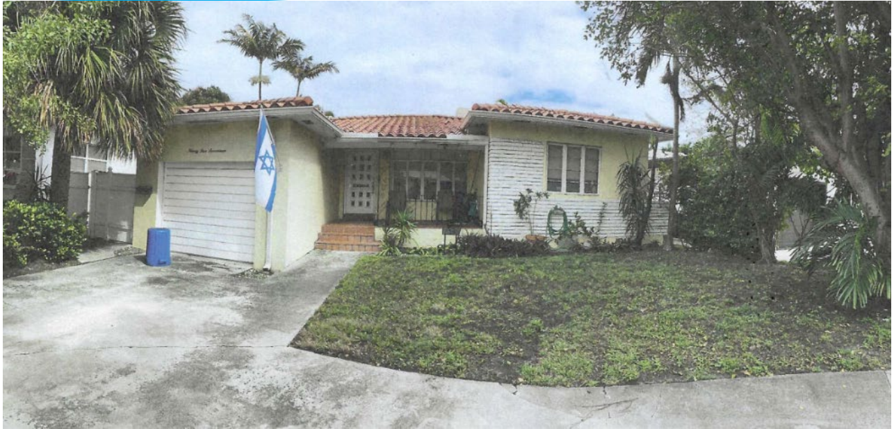
West Elevation of 9517 Byron Avenue
