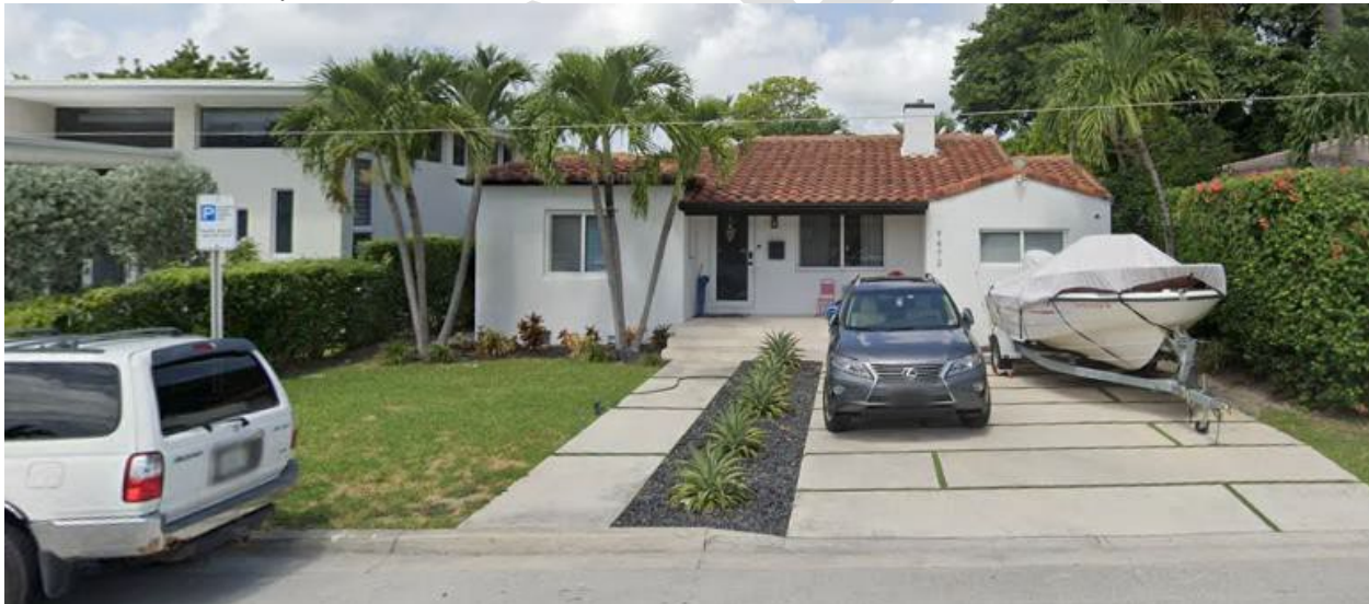
West Elevation of 9472 Byron Avenue
