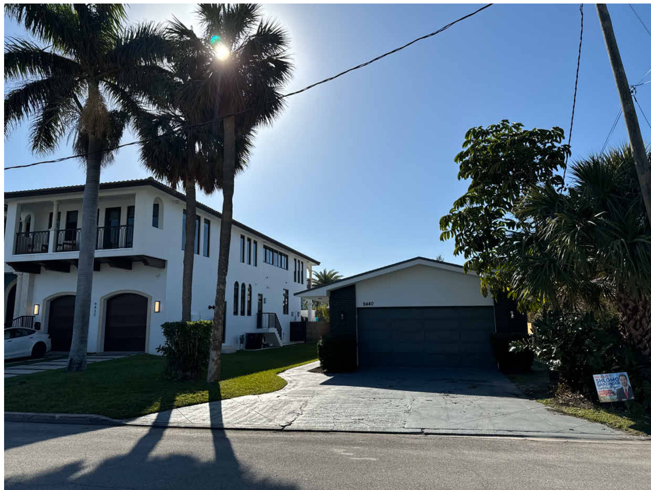
EXISTING HOUSE TO THE SOUTH
