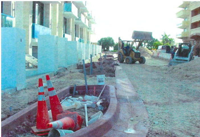
Pictured is 95th and Collins to bulkhead
