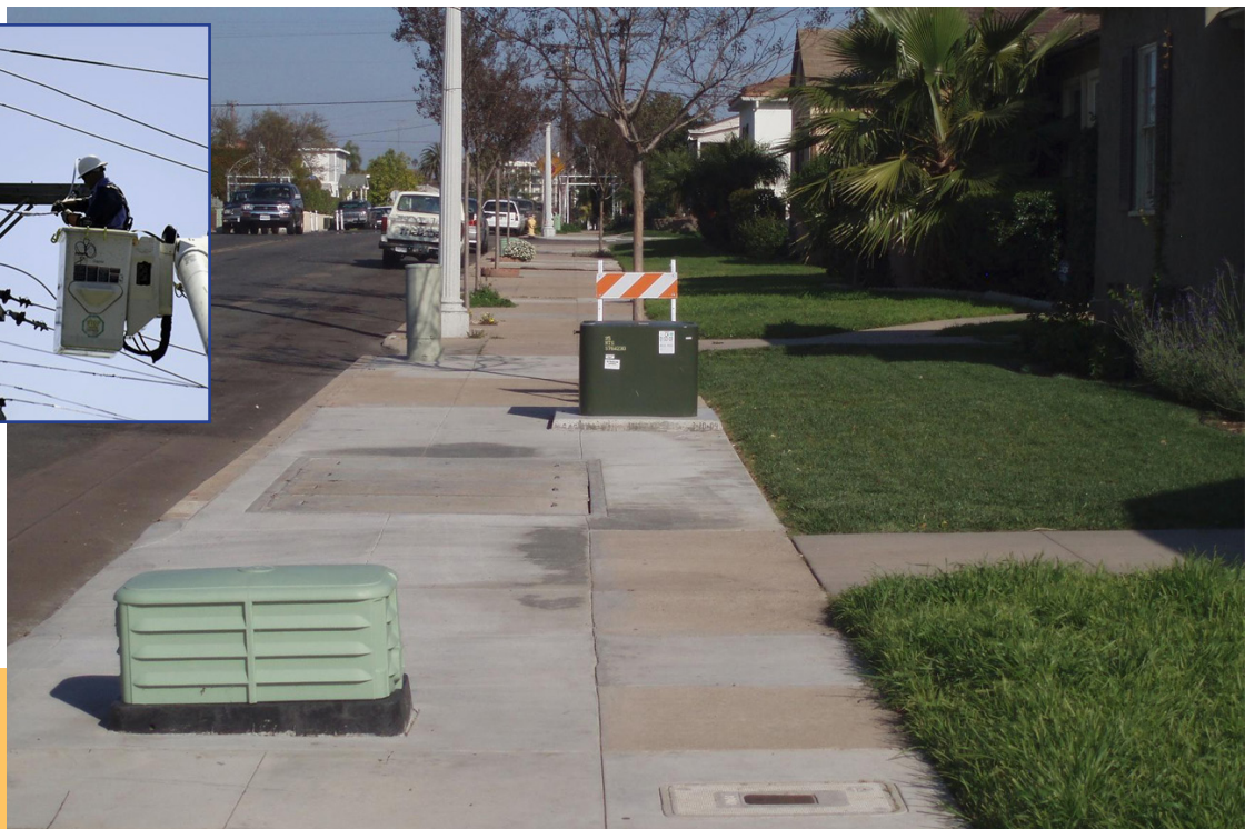
Overhead lines and poles (inset) would be replaced by above-ground access boxes located on property lines (shown at right)
